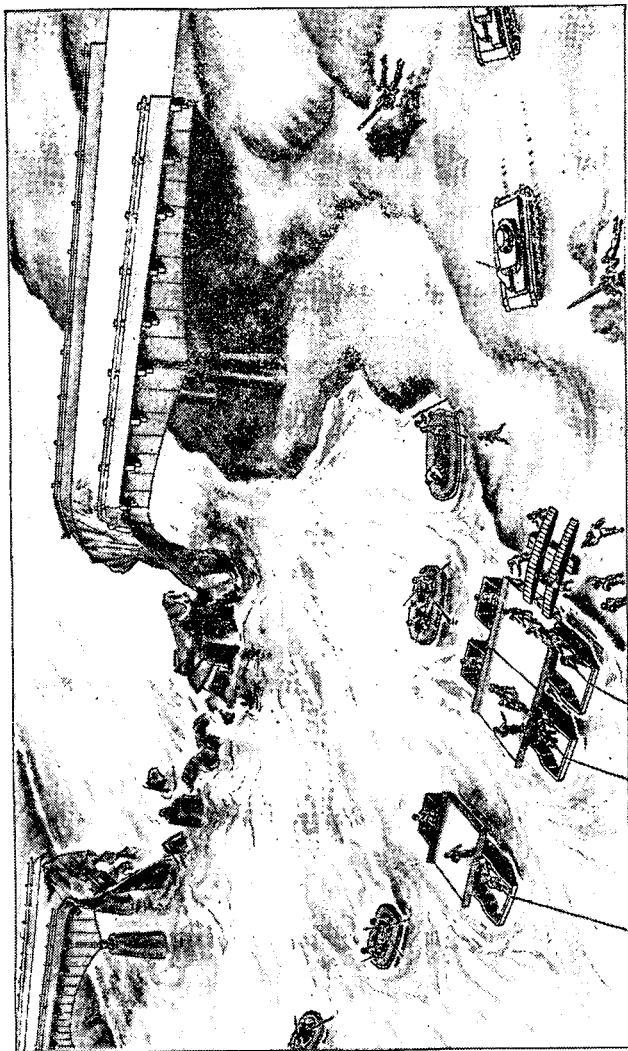
FIGURE 59.—Demolition should be of such extent that it will take the enemy longer to repair the bridge than to construct a new temporary bridge or ford.
