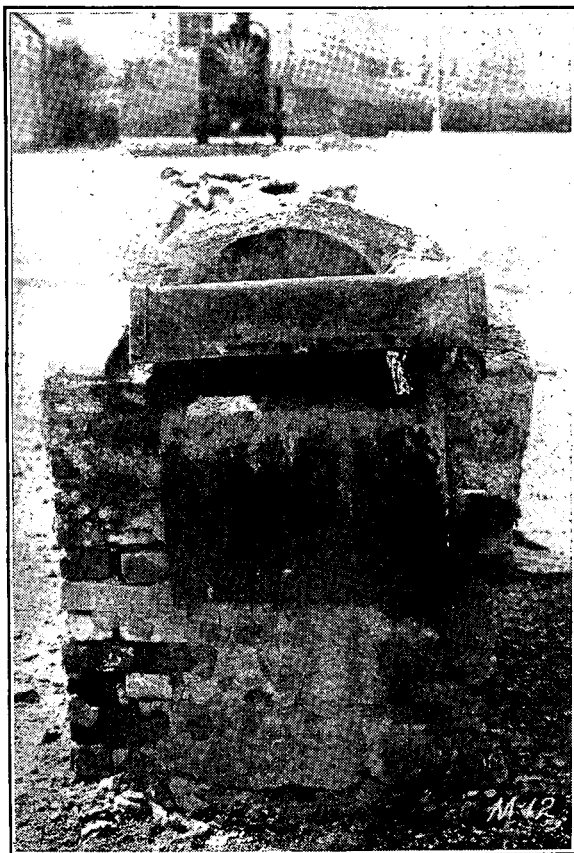
FIGURE 19.—Incline plane incinerator, end view.
