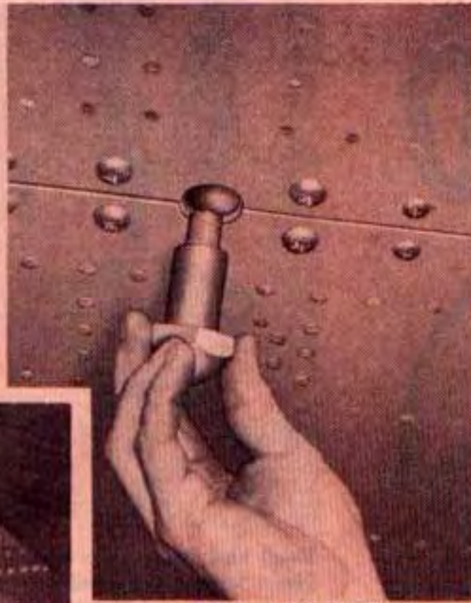
E729 WING OUTER JACK FITTING
