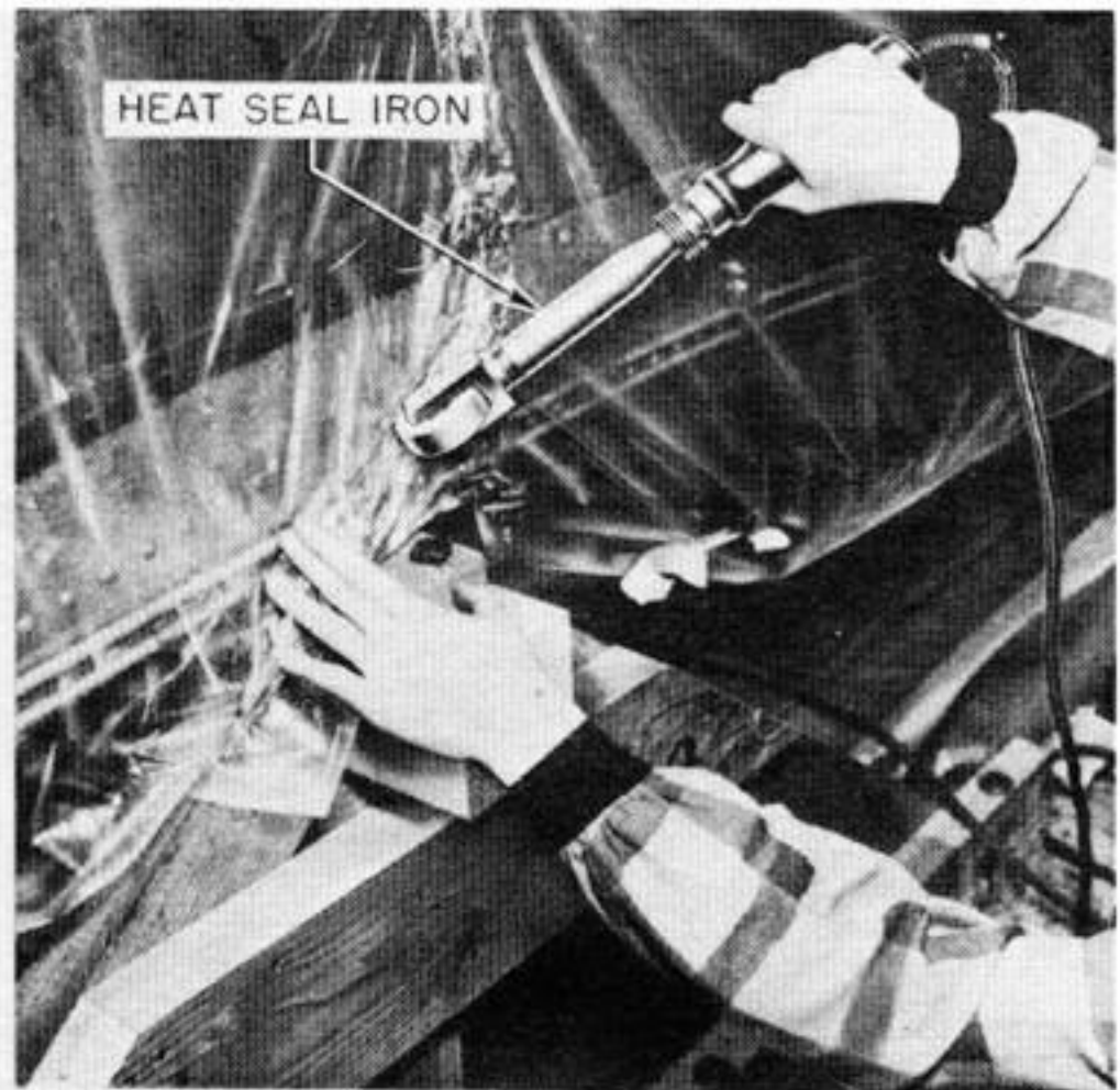
JOINING SEAM WITH HOT IRON
