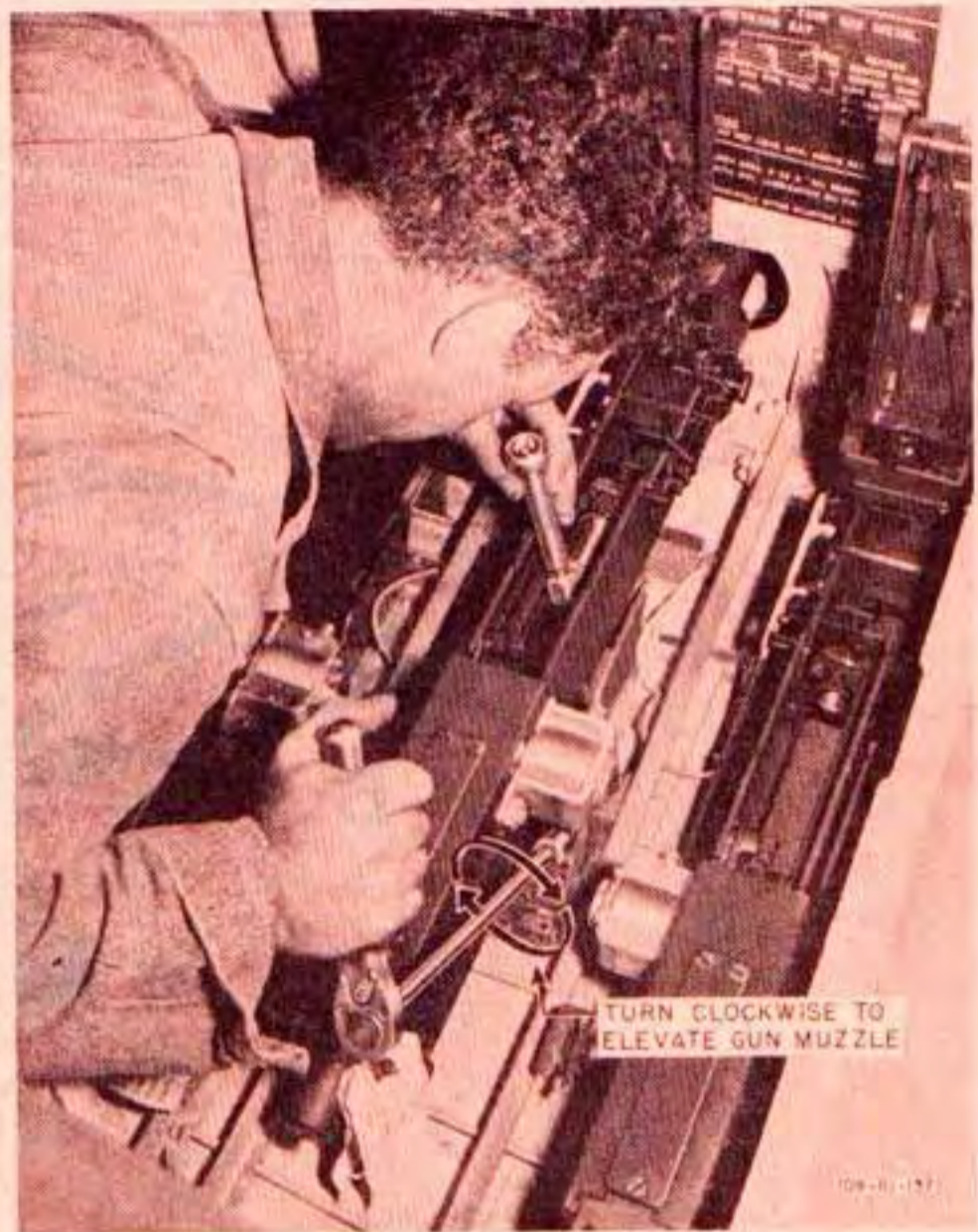
Figure 441—Adjusting Gun in Elevation
