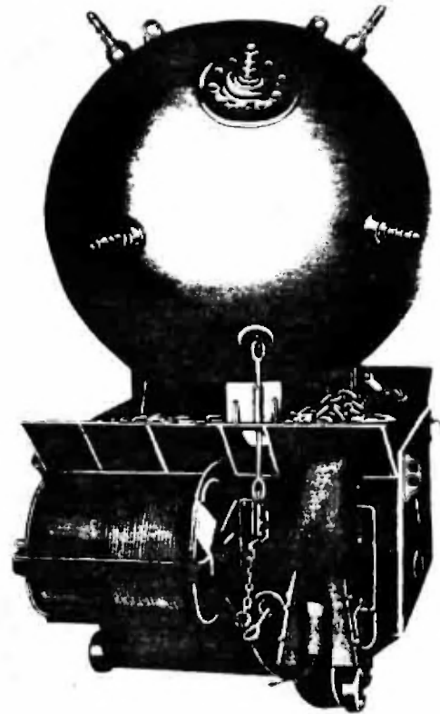
Figure 13 - EMC II Mine with 20-ft. Mooring Chain
