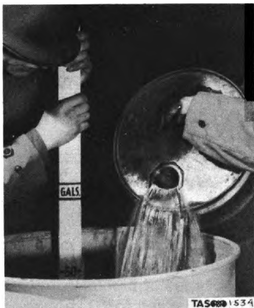
Figure 33. Measuring Ordinary Gasoline into Mixing Drum.
