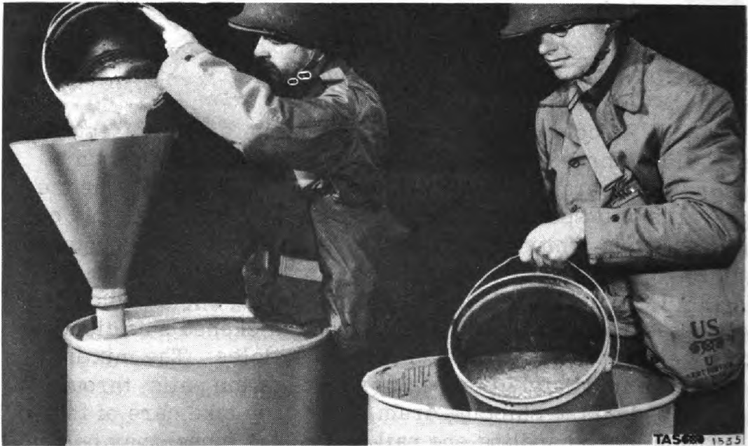
Figure 35. Transferring Newly Mixed Fuel from Mixing Drum to Shipping Drum, Where It Will "Age."
