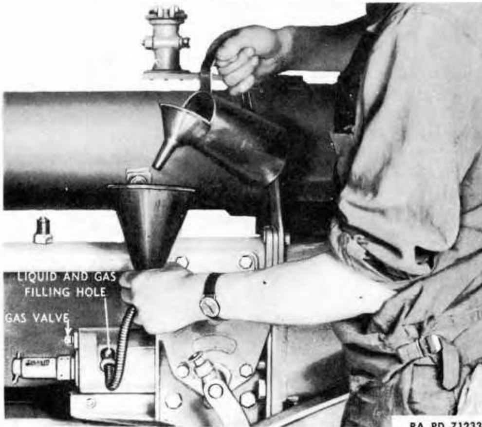
Figure 60 — Filling Rammer Cylinder with Liquid
