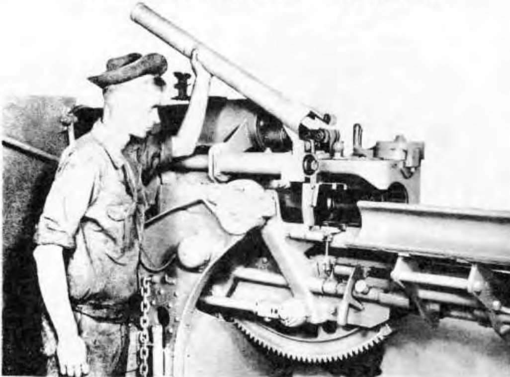
Figure 40 – Unfolding Rammer Guard
